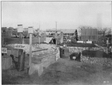
Fig. 1. This and 2 pages follow present view of the factory full application constructed at Millard Street Pumping Over, Butte, Mont.
